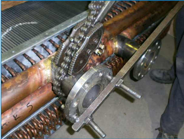
Installing screw-on flange
