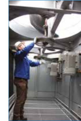
Fan drive system easily accessible while standing
