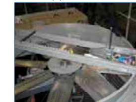
Mechanical equipment removal*
