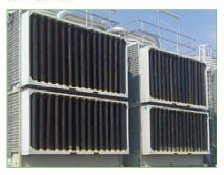
FXVT closed circuit cooling towers use **quiet and low kW axial fans**, but to reduce noise even further, you can extend your FXVT with sound attenuation:
