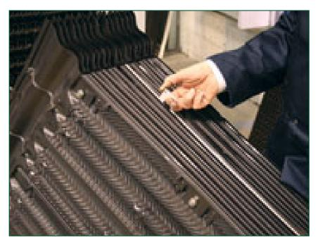
BACross<sup>®</sup> bundles include <u>BACross<sup>®</sup> fill sheet packs</u> with an handle to hang the bundles on the fill support.
