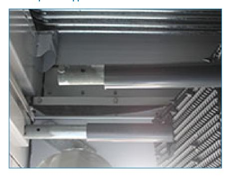
The use of telescopic fill support beams facilitates the replacement of the fill sheets.
