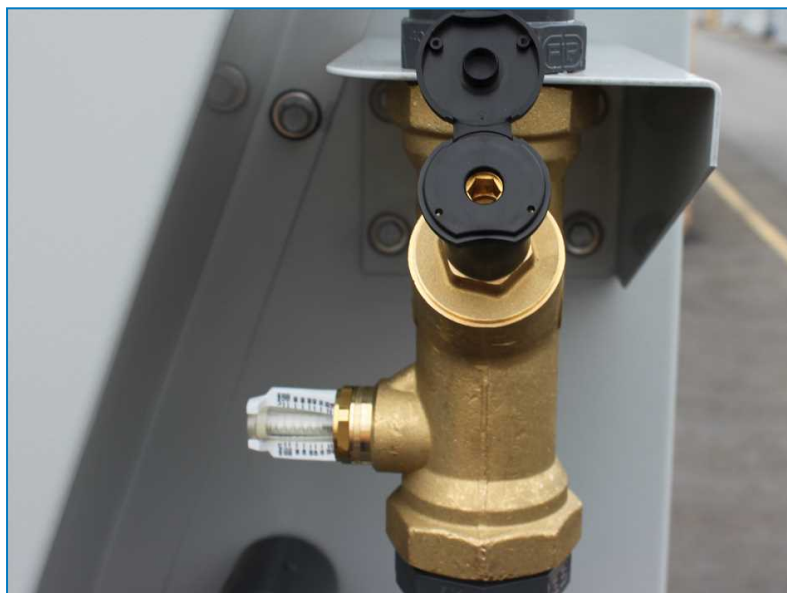
Water flow adjustment screw
